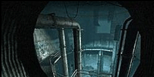
2. The Drains/排水溝
